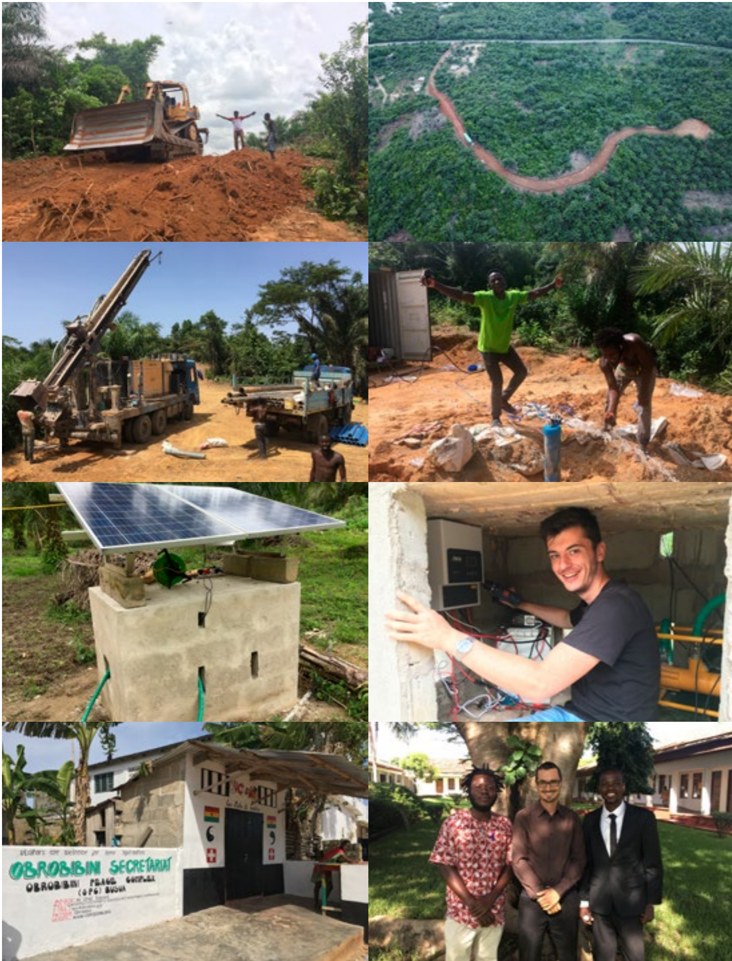
Construction of the access road (top), water drilling (upper middle), first solar plant (lower middle), office work (bottom left) and Executive Board before the presentation at the University of Ghana (bottom right)
