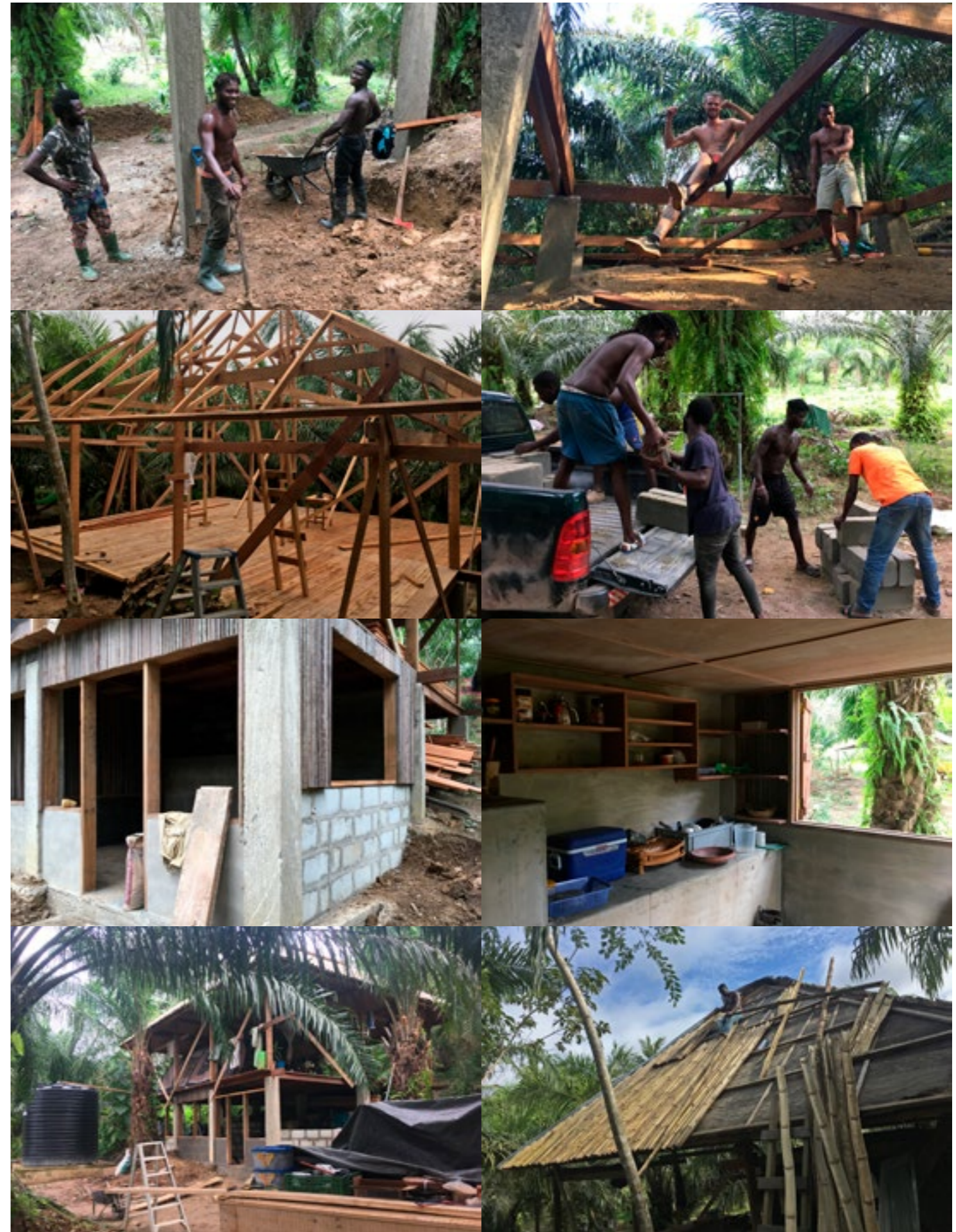
Impressions of the construction of the wooden platform, which has meanwhile developed into a three-storey building with kitchen, storeroom, platform and mass sleeping area
